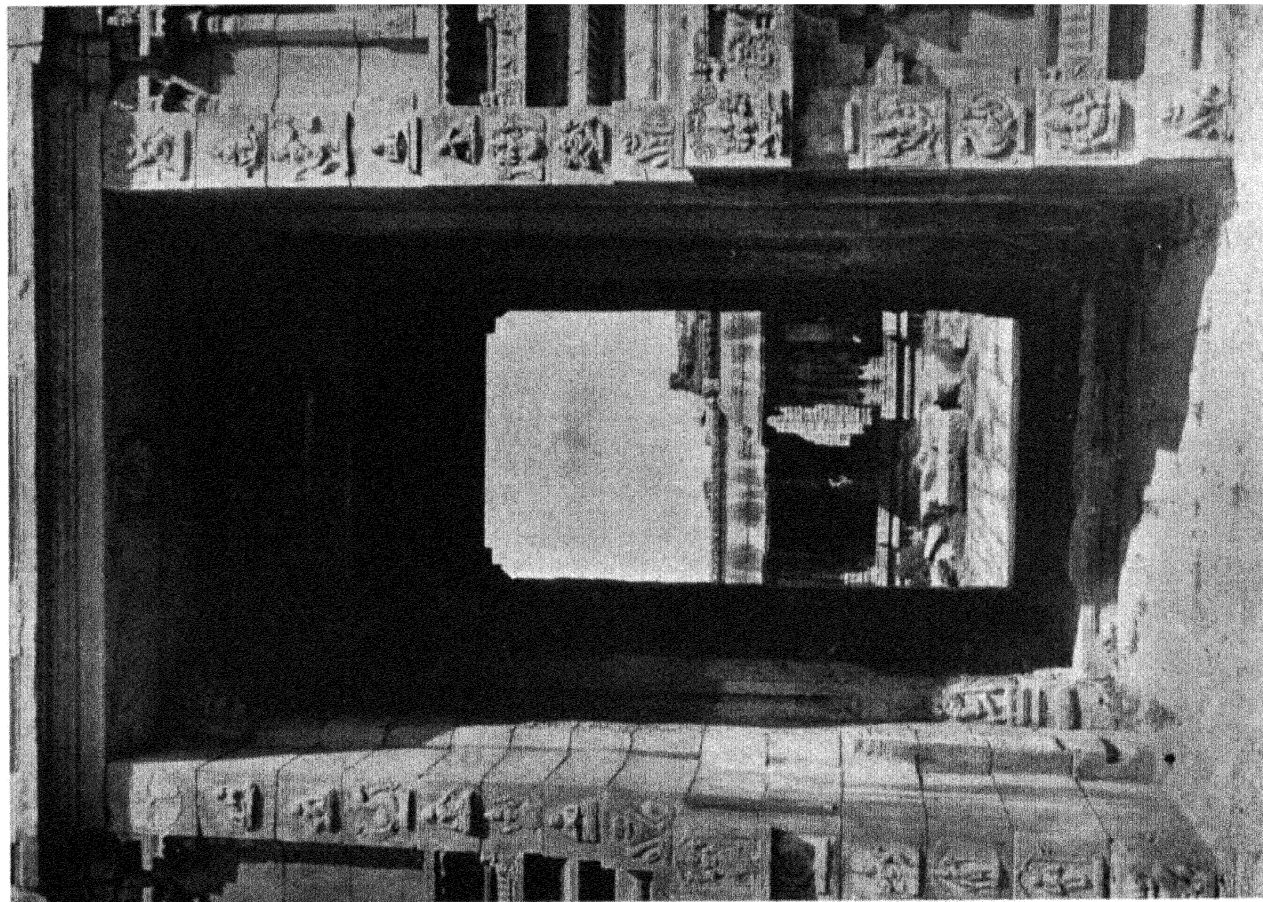
b. THE SAME: SHOWING PILLARS IN THE ENTRANCE REMOVED AND IRON GIRDERS FIXED IN PLACE OF SAME.
