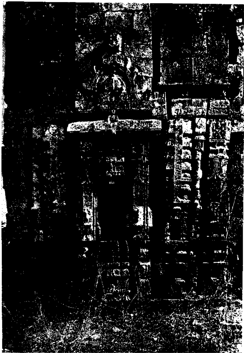
Bāṛa consisting of pabhaga , jangha and baranda in a ruined Temple near Kotitirtha, Bhubaneswar
