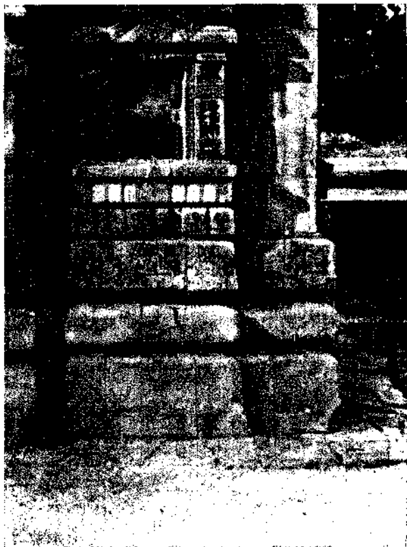
Pabhaga , consisting of three mouldings, Parasurameswar Temple, Bhubaneswar
