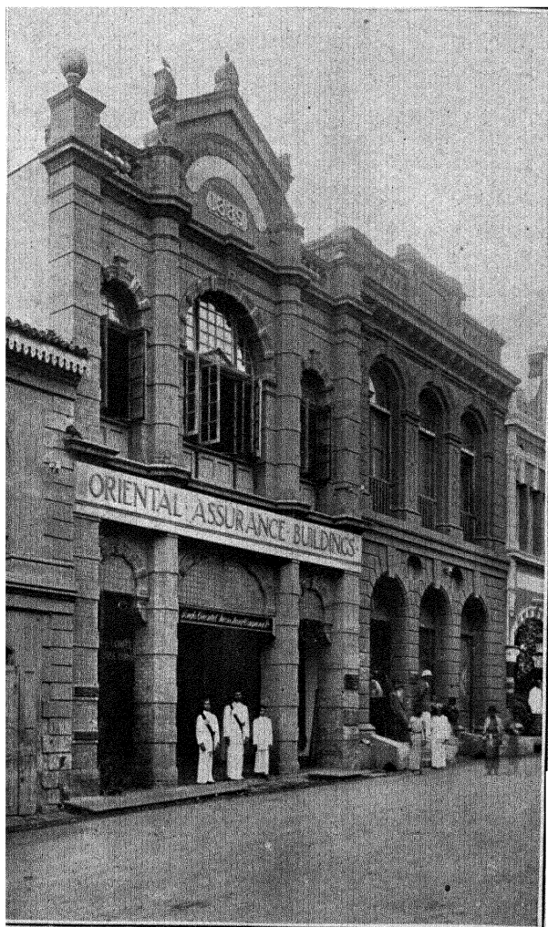
ORIENTAL ASSURANCE BUILDINGS, COLOMBO.
