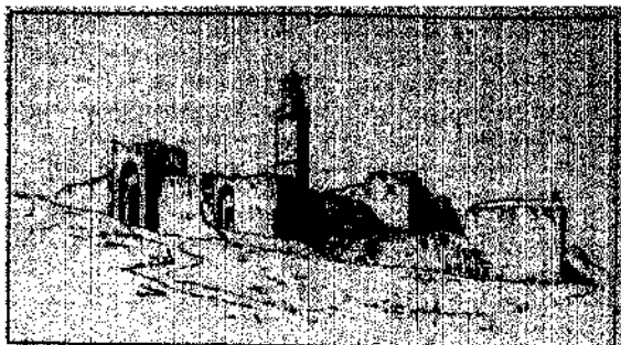
NEBY MOSA, LOOKING TOWARDS THE NORTH-WEST.
