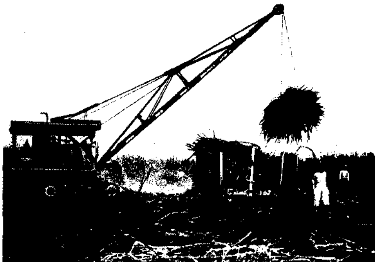
Mechanical cane loader at work on an Hawaiian sugar plantation
