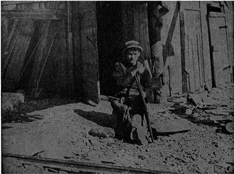
FIG. 2. — Splitting slate. (H. Ries, photo.)
