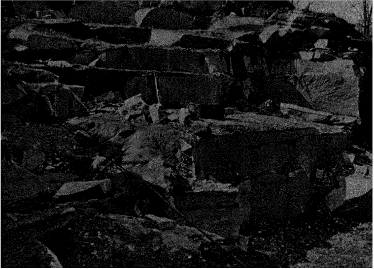
PLATE XXIX, FIG. 1. — Granite quarry, near Woodstock, Md., showing horizontal joints. (T. L. Watson, photo.)
