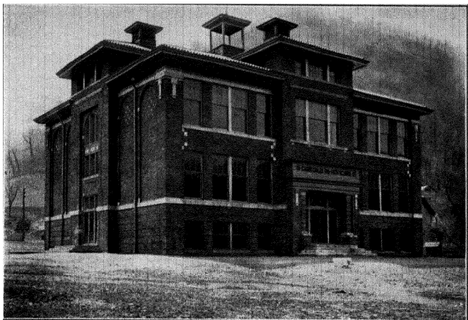
New building, District High School, East Bank, Kanawha County, W. Va.
