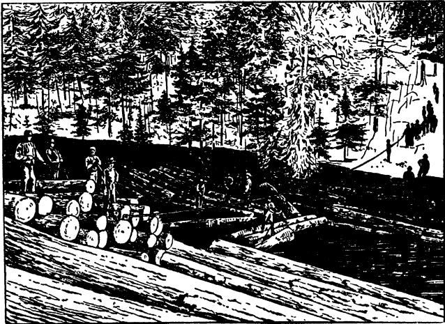
FIG. 54.—Lumbering in Canada. Logs dragged over the snow are being fastened together to form rafts.
