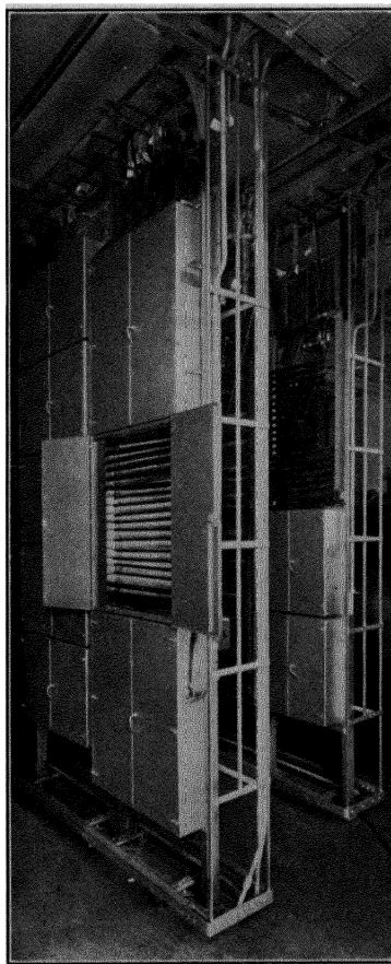
FIGURE 36. Aluminum paint on telephone exchange equipment. (Courtesy of Bell Telephone Laboratories.)
