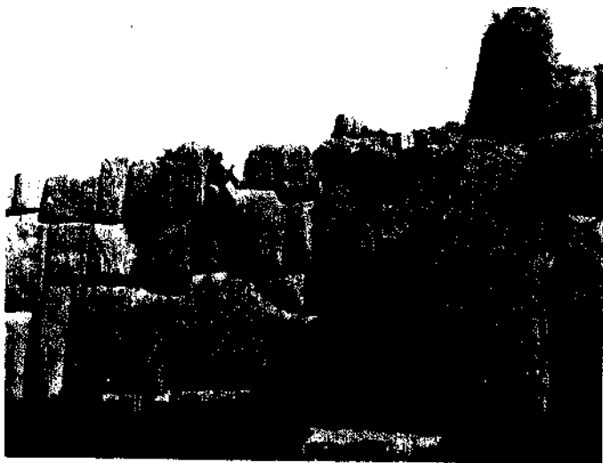
FIG. 60. A detail of the lowermost of the three northern walls of the Fortress of Sacsahuaman. The large stone on the right weighs about 150 tons.
