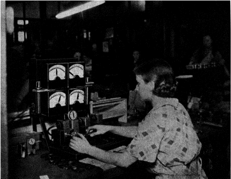
FIGURE 39. A practical operation: checking the dimensions of shafts. Four electric gauges magnify a variation of 0.0001 inch to give a half-inch movement of the instrument pointers. (Courtesy General Electric Company.)
