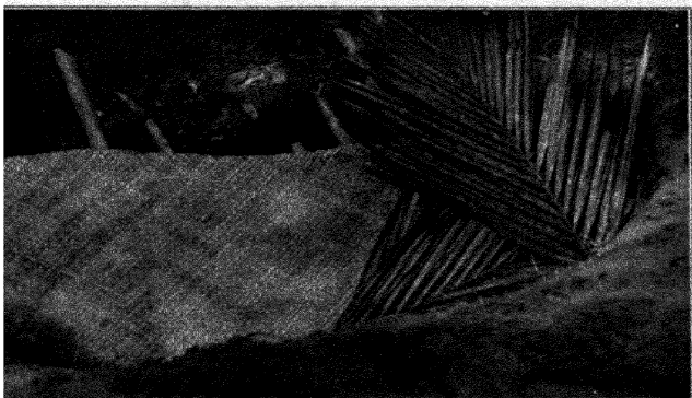
CLOSING THE SIDE CHAMBER WITH BAMBOO, LEAVES AND MATTING
