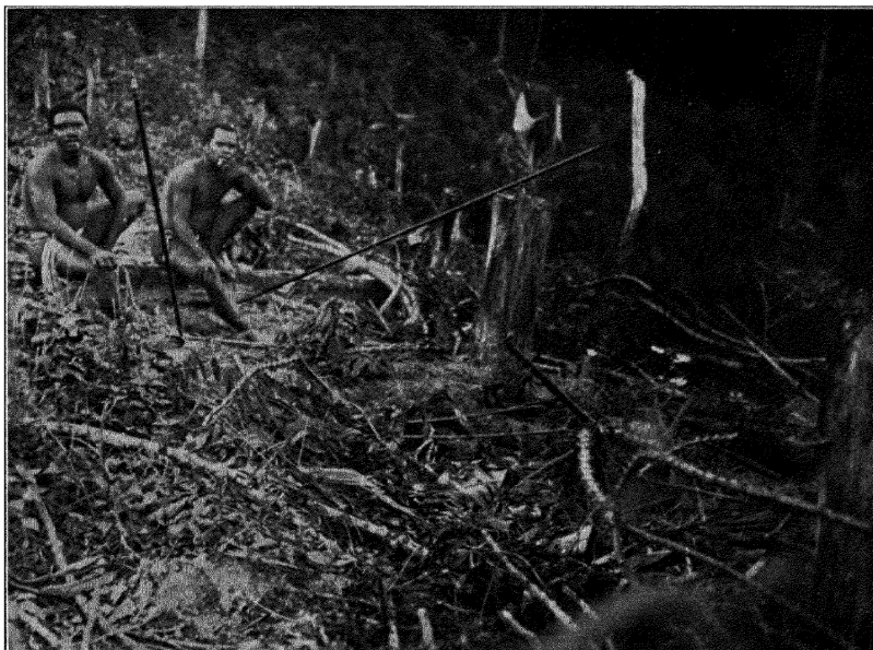
THE DAMAGE WAS SERIOUS (p. 84)
