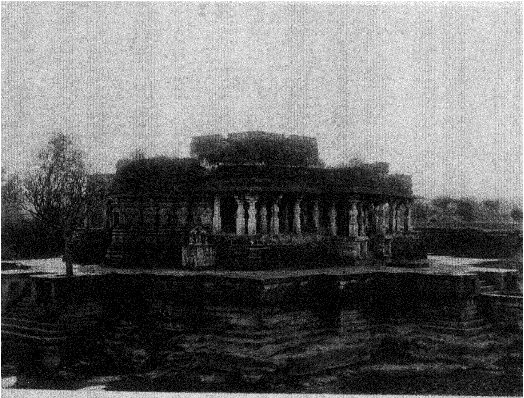
(b) KHANQAH TEMPLE AT BIR: GENERAL VIEW
