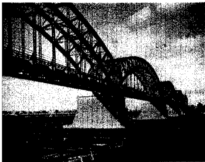
VIII.—WARSAW: NEW RAILWAY BRIDGE ACROSS THE VISTULA
