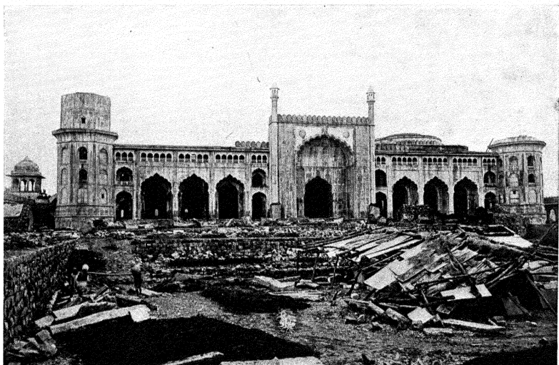
GREAT MOSQUE UNDER CONSTRUCTION (BHOPAL).
