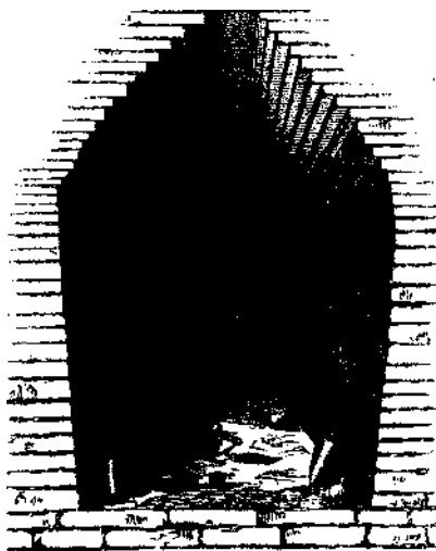
Brick vault at Mugheir.
