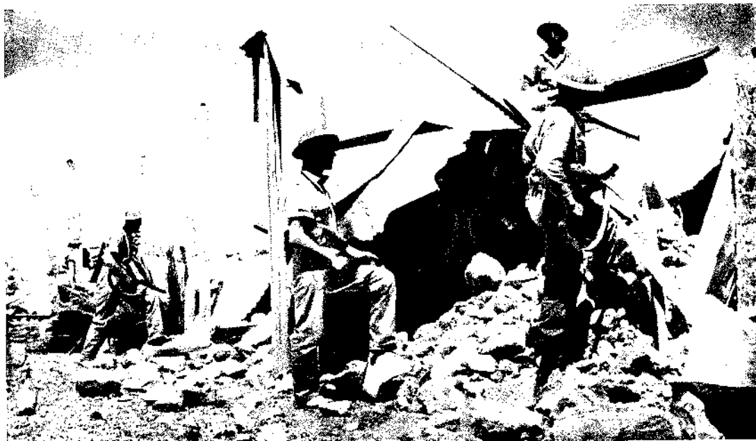
Pierce shelling from British artillery has reduced an Italian fort to a broken mass of masonry. This picture from the Western Desert shows our infantry moving in to occupy the ruins.
