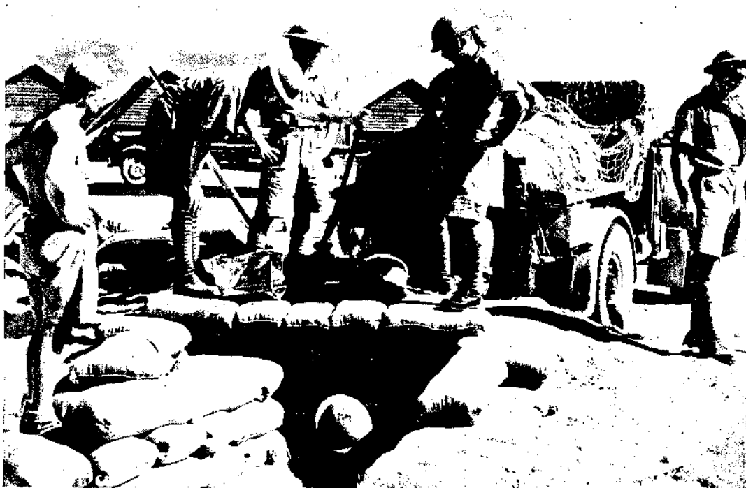
In the barren land where the Army of the Nile was operating, supply of water was a problem of major importance. It was overcome by the sinking of deep tanks, one of which is shown being filled.
