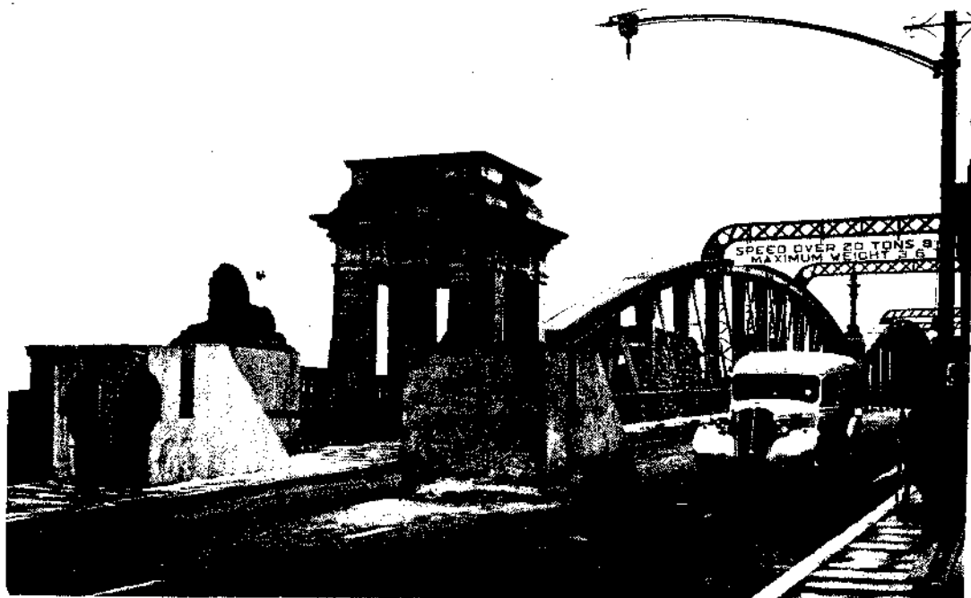
This bridge in the south of England has its double guard of sentry, on the right, and strong concrete road blocks. Every town and village has its own effective method of meeting the threat of enemy invasion.
