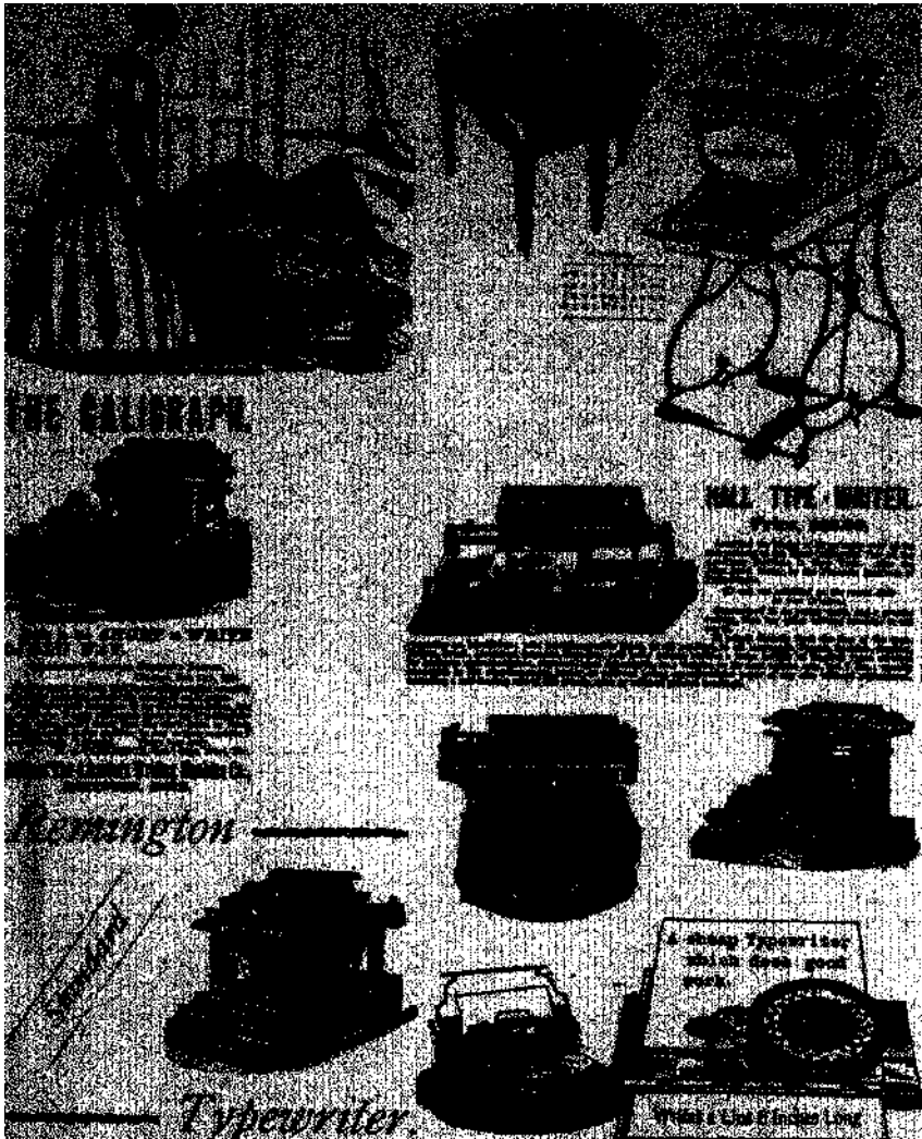
TOP: Union carpet sweeper, 1865; one of the first typesetting machines, 1857; typewriter on sewing-machine stand with treadle-operated spacer. SECOND ROW: The calligraph typewriter, 1885 ; the Hall typewriter of 1885. Note the price was $40 and that it required no ribbon and had interchangeable type to write Sanskrit, Japanese, Armenian, Greek, and German. It would operate from a roll of 500 sheets of paper! BOTTOM : The Remington Standard of 1890; the National typewriter and the Yost typewriter of the 1890s; the Hammond, circular-keyboard typewriter of 1888; Child's typewriter of 1892, priced at $2.50.
