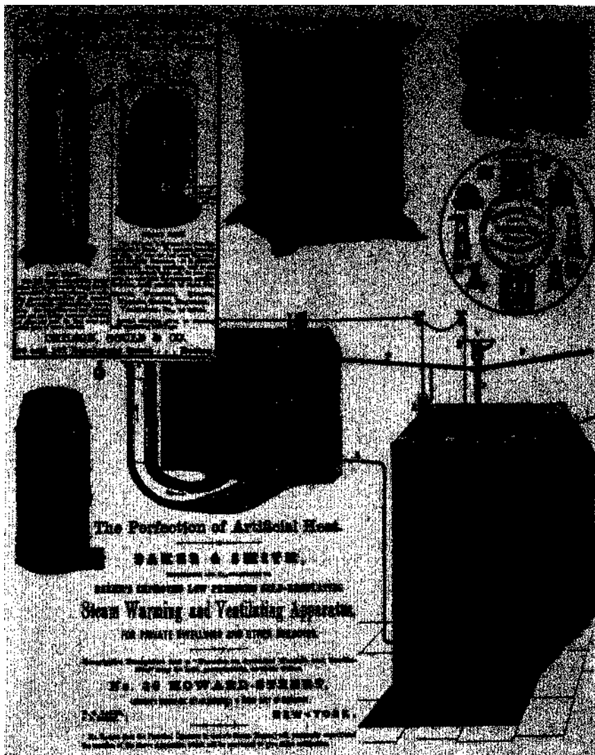
TOP : Advertisement by Chilson, Gould & Co., Boston, 1850. The Trio stove pictured is built in the form of a huge tuba. The same basic design was used in the portable furnace, also pictured. Steam radiator of 1850s with ornate cast-iron grille work on four sides, iron base, and marble top. Wood-burning furnace of 1865. Many of these were used in cottages and homes of the Midwest and Northwest. Advertisement of Prouty & Co., stove dealers of Boston, 1850. BOTTOM: Enclosed furnace for installation in cellar, 1856; advertisement of Baker & Smith, featuring their steam warming and ventilating apparatus. This advertisement of 1850 features indirect steam heating, considered a modern invention.
