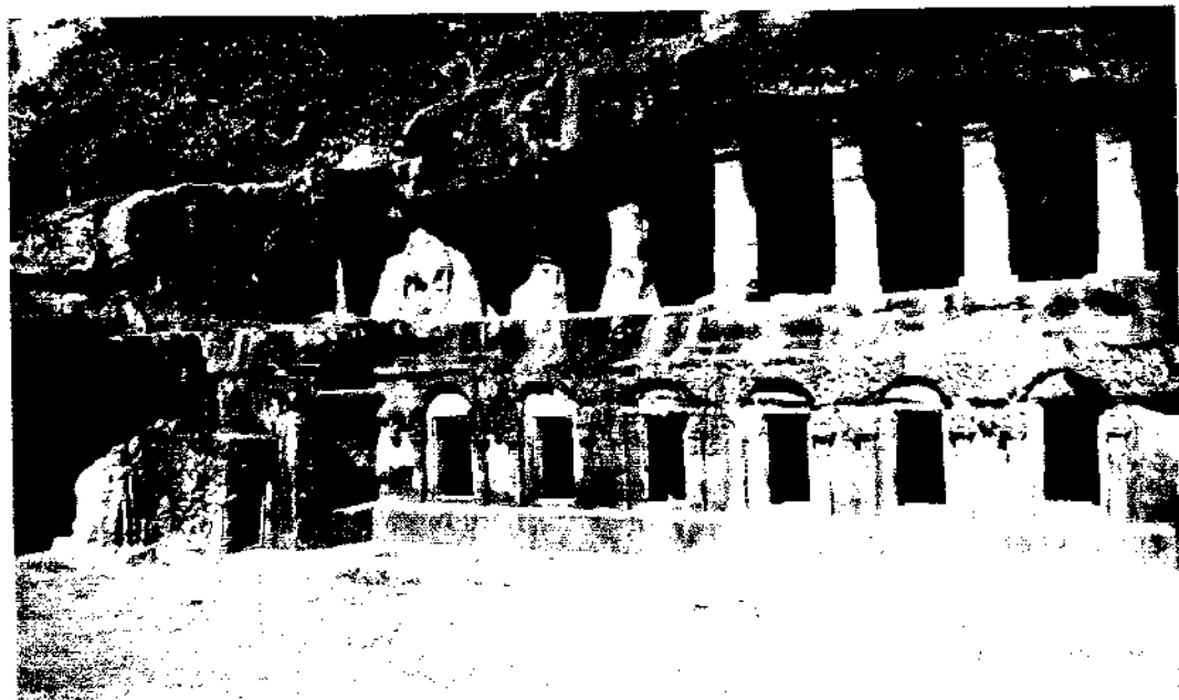
Rani Nur Gumpha —General View Left Portion of the Central Wing, Illdaygiri, Puri district
