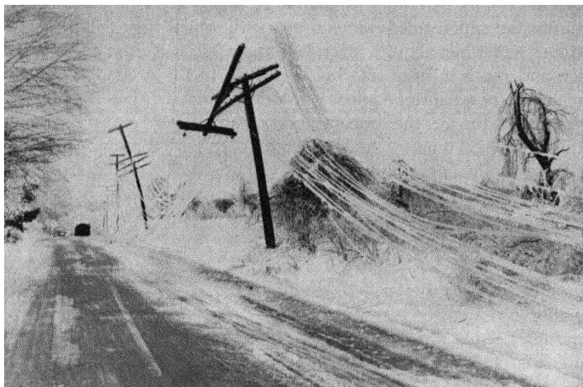
Fig. 67. Telephone Lines and Trees Broken by the Weight of Glaze Ice Near Mount Freedom, New Jersey, January, 1953. Damage to communication lines becomes severe when the diameter of ice covering the wires exceeds \frac{3}{4} inch. The Bell Telephone System suffered damages of $8,000,000 from a single ice storm in January, 1951. Courtesy, Southwestern Bell Telephone Company.
