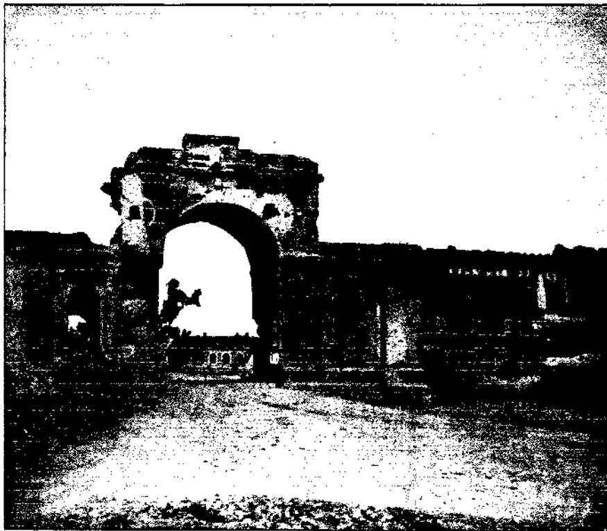
EXTERIOR VIEW OF THE BAILEY GUARD GATE.
