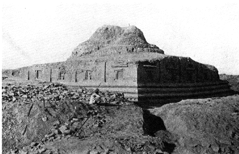
STUPA I AT MIRPUR-KHAS, AFTER EXCAVATION
