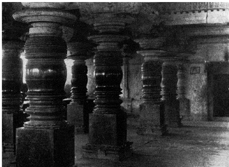
INTERIOR OF TEMPLE AT ANNAVATTI
