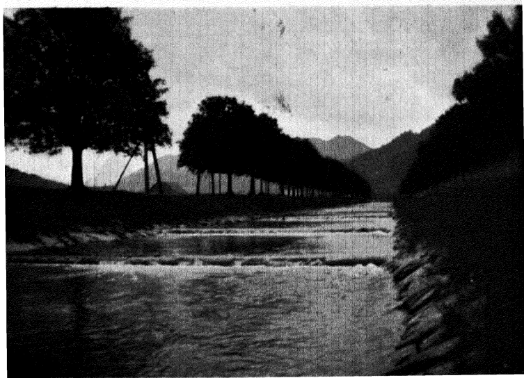
FIG. 39.—CHECK DAMS IN RIVER TO PREVENT EROSION OF BED, SWITZERLAND
