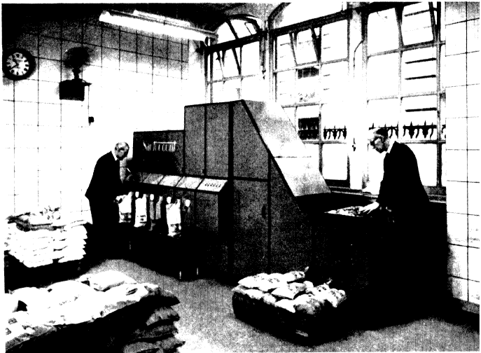
An automatic coin-sorter at work in a bank bullion department
