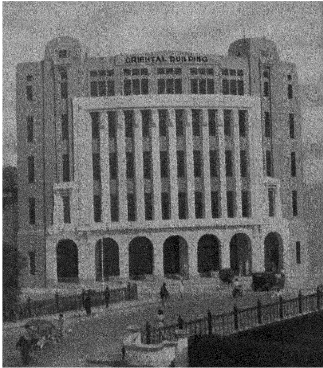
ORIENTAL BUILDING, KUALA LUMPUR
