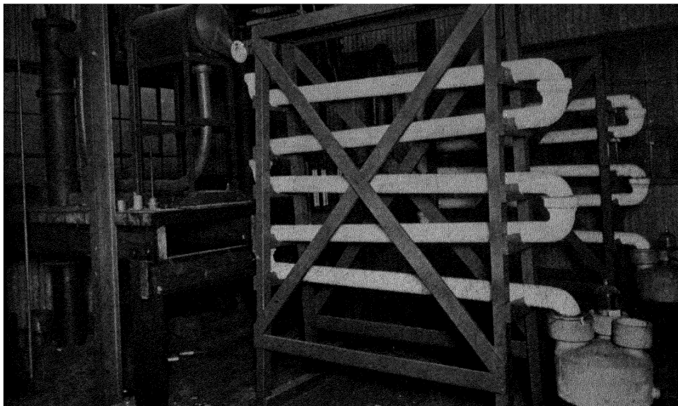
Fig. 4.—AMMONIA OXIDATION PLANT SHOWING CONVERTER AND SILICA COOLER.
