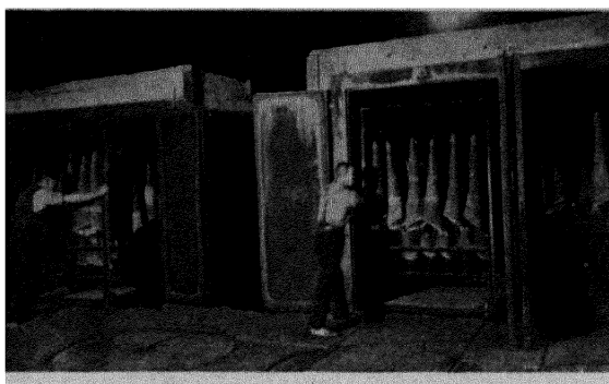
Fig. 8.—" DRY-HEAT " VULCANISING CHAMBERS. Showing batches of waterproof " waders " being loaded in ready for the vulcanising process.
