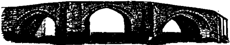
BOW BRIDGE AS IT STOOD BEFORE ITS DEMOLITION IN 1839. (From a print dated 1831.)
