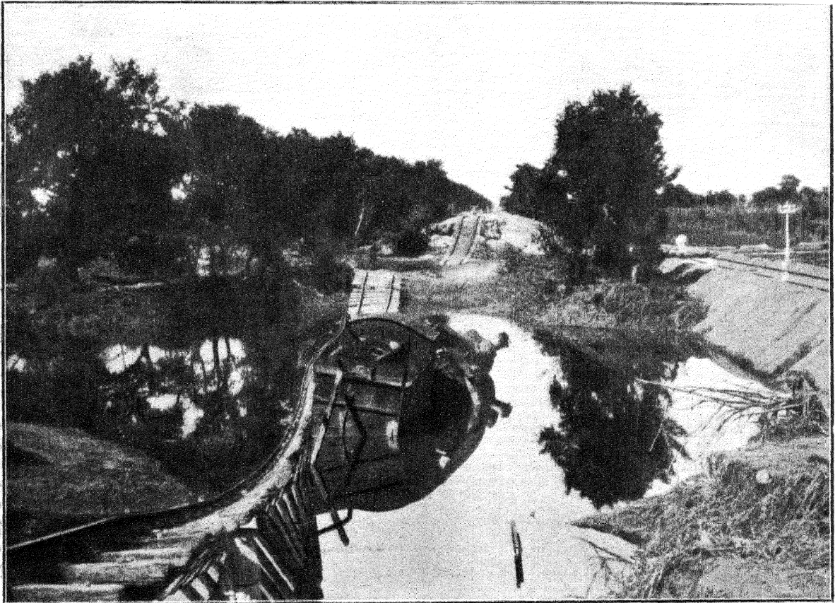
Engine in breach near Lhaksar, Oudh and Rohilkhand Railway, during the floods.
