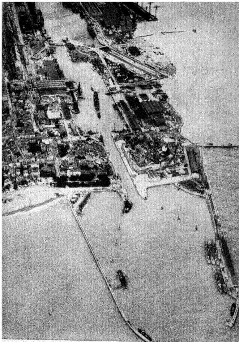
Oblique air view of the St. Nazaire docks, taken from south. For identification of main features, see line drawing, Figure I (page 81).
