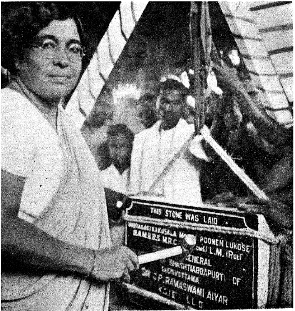
Foundation Laying of the Maternity Ward, Nelumangad District Hospital
