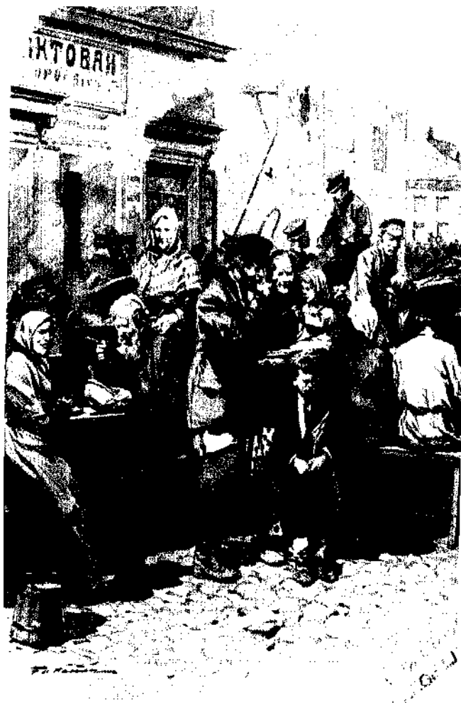
AN OPEN-AIR KITCHEN
