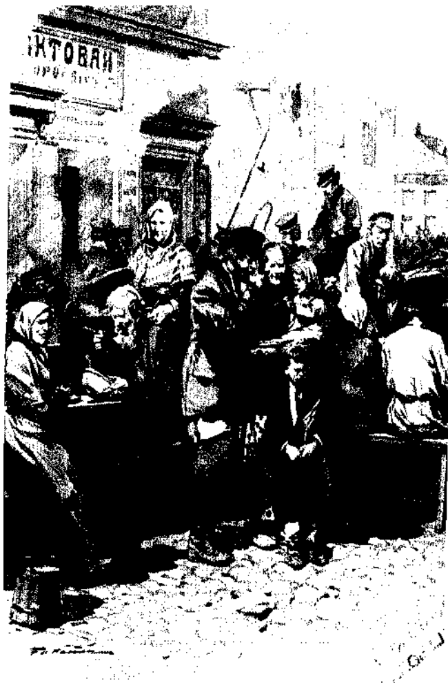
AN OPEN-AIR KITCHEN
