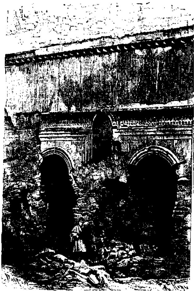
52 RUINED PALACE AT FIRUZABAD. CENTRAL HALL,
