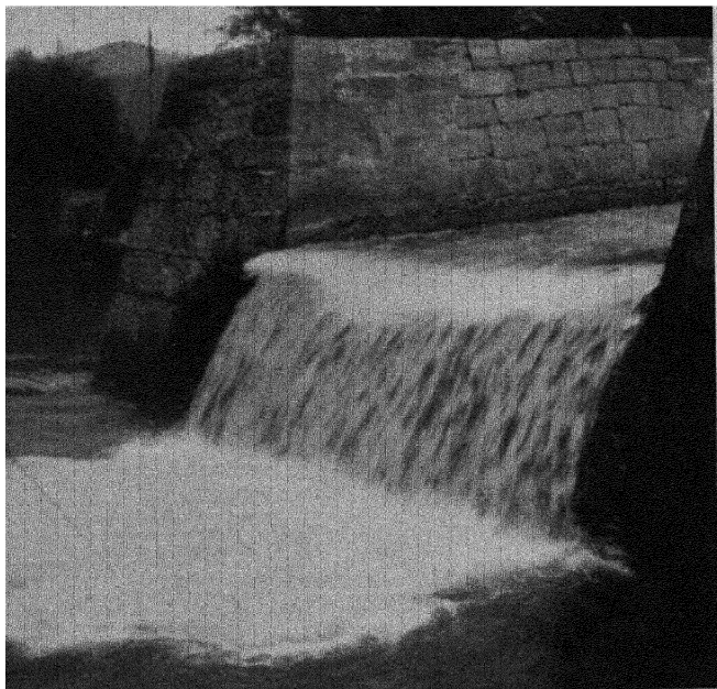
FIG. 1.—A Roll Wave leaping the Outfall of the Grünbach Conduit.
