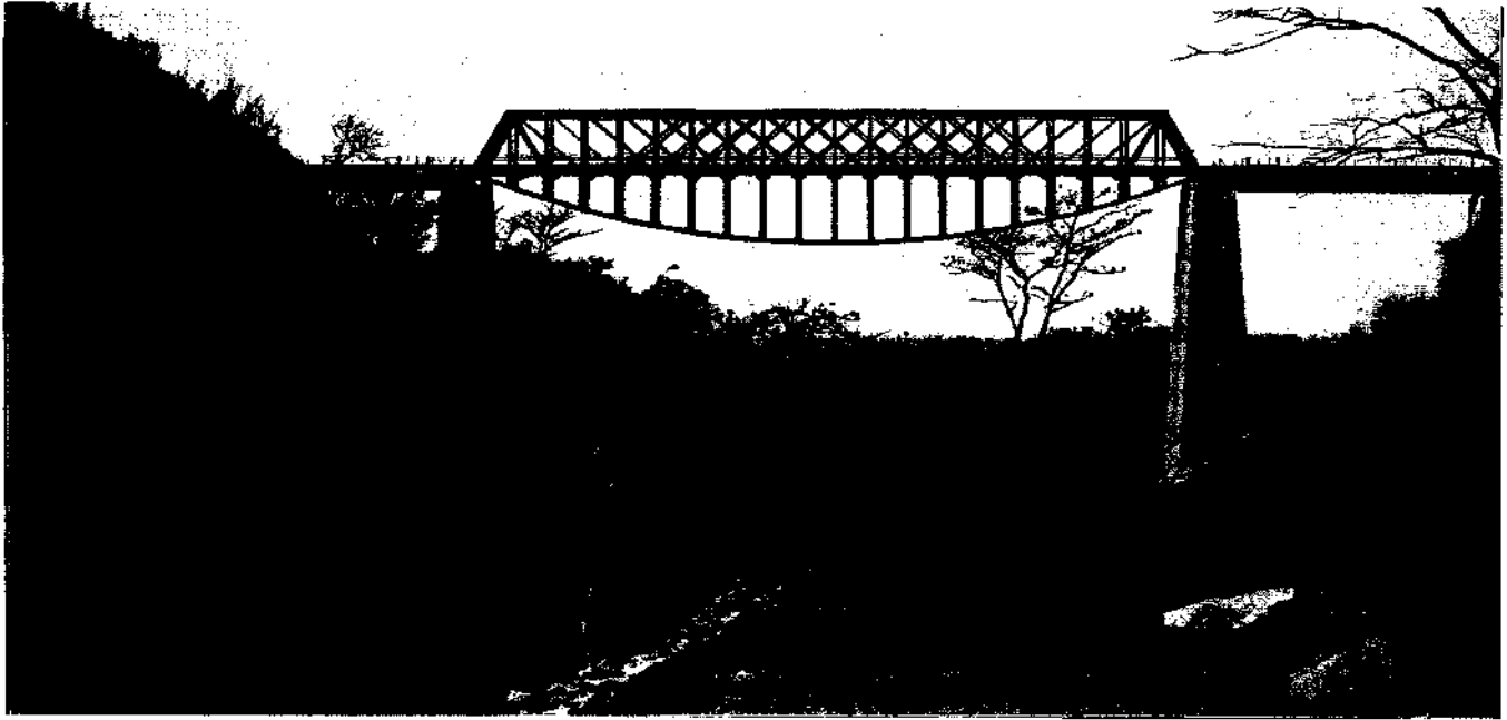
Dhorabhavi Bridge, Guntakal-Bezwada Section—250 span strengthened by underhung bowstring.
