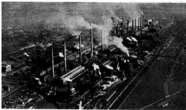
AMMONIA WORKS AT MERSEBURG
