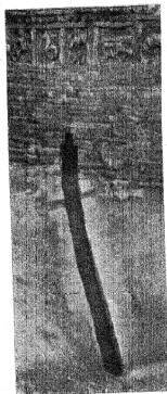
(e) Paharpur, Main Temple: Drain under First Terrace Verandah.
