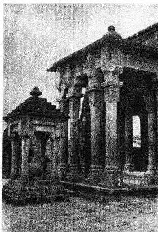
(a) Kaugra : Baijnath Temple, after Removal of Plaster etc., from Columns.
