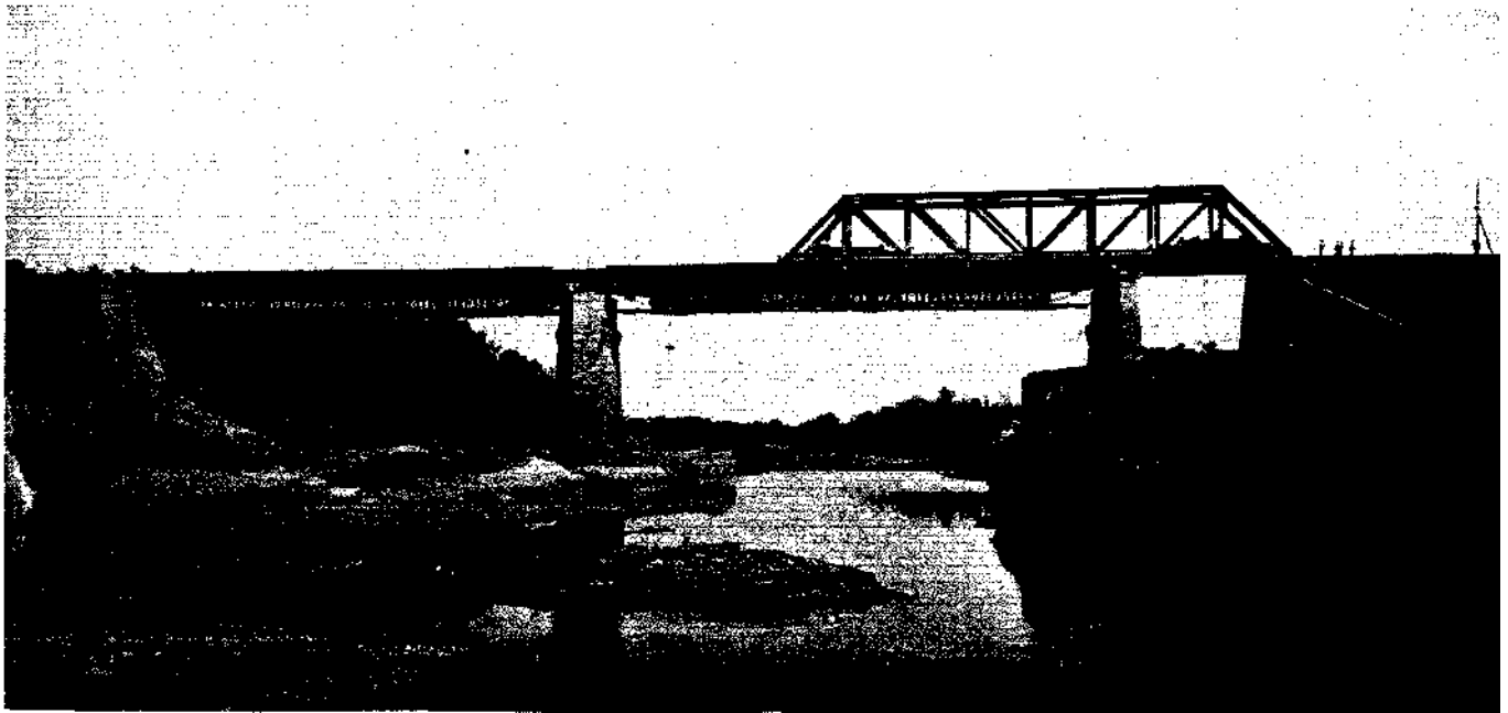
Reconstruction of Johilla Bridge (New Span being launched)
