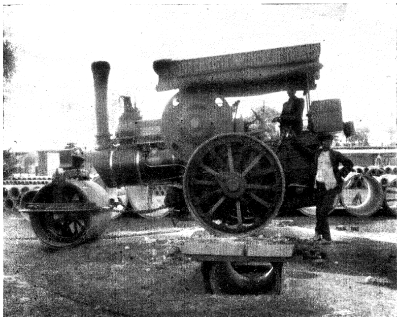
HUME PIPE UNDER HEAVY LOAD TEST
