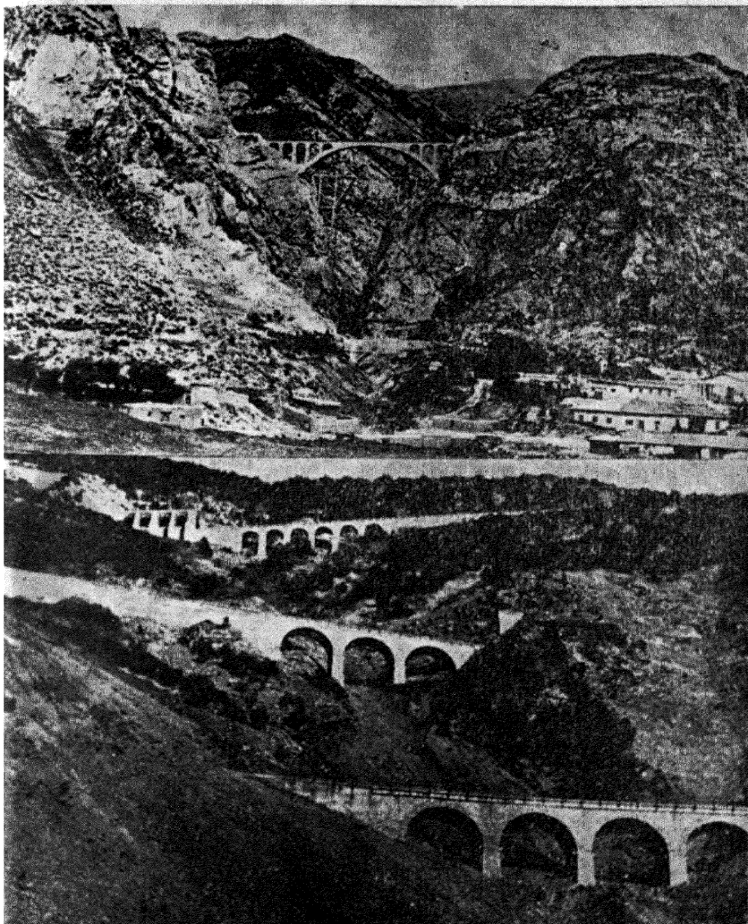
Transcaucasia: pont de Verek. The Verek Bridge - One of the engineering masterpieces of the Transcaucasian Railway.
