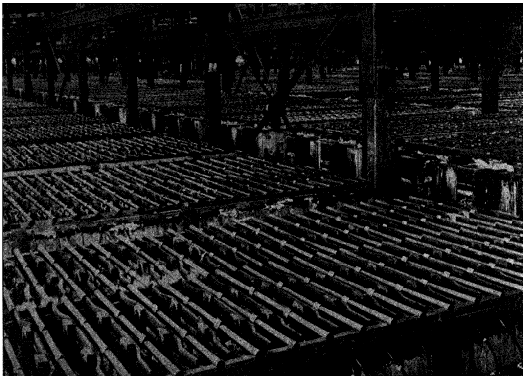
Figure 264. Refining Nickel by Electrolysis (Courtesy of the International Nickel Company)
