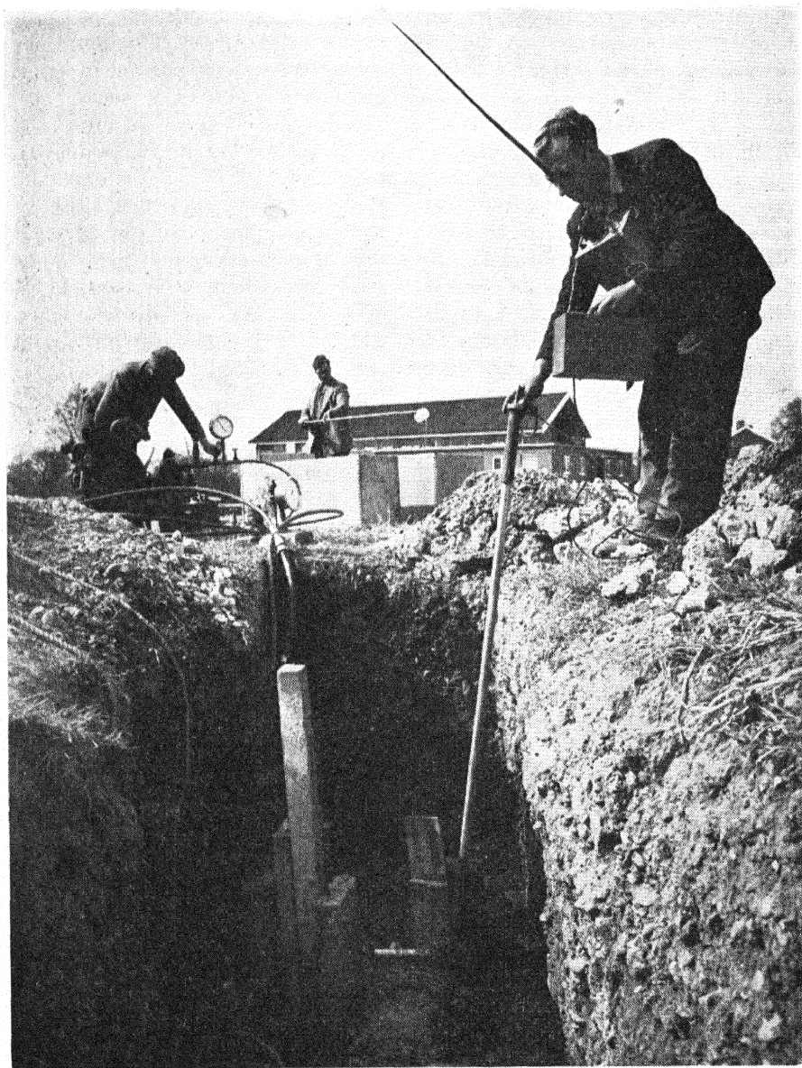
Testing for leaking mains with a Geiger counter
