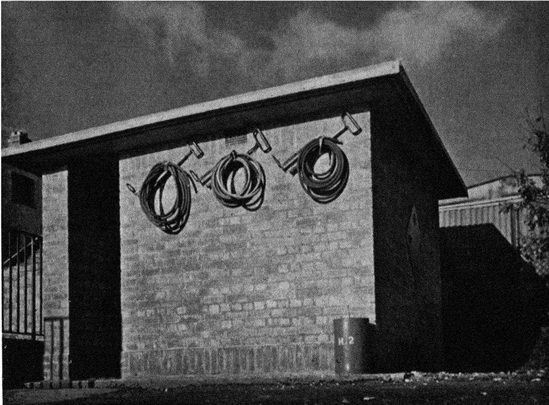
Brick and concrete wardens' post with stirrup pumps.
