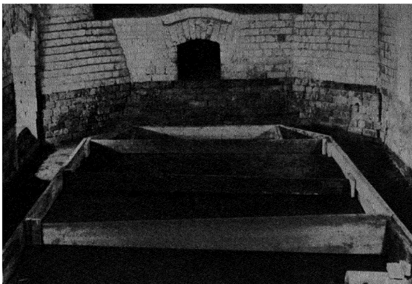
FIG. 108. Ramming a basic hearth.
