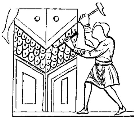
TILING WITH WOODEN SHINGLES.
