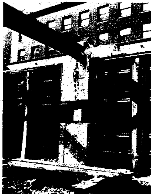
The primitive form of skeleton construction used in the Home Insurance Building, showing that the outside walls were supported by the cast iron columns and lintels.
