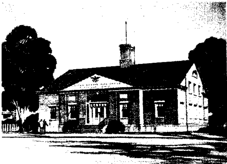
A typical Post Office designed in Washington under supervision of a board of advisory architects—Modernized Classic.
