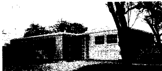
A Prefabricated House as built by General Houses, Inc.; steel frame, asbestos-cement board.
