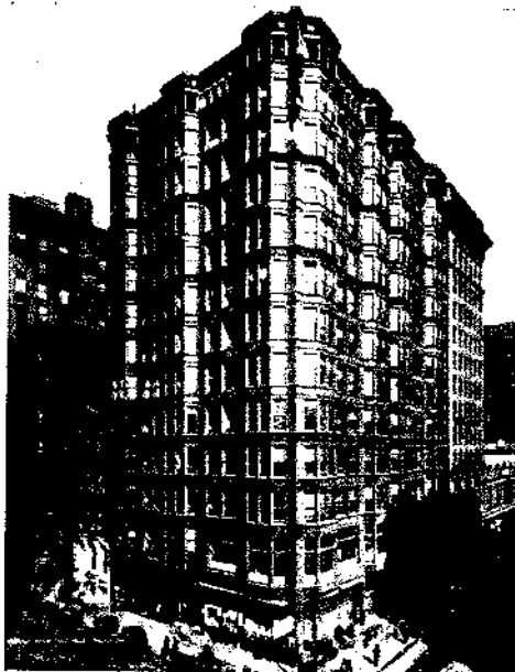
The Tacoma Building, Chicago, Holabird and Roche, architects, built in 1887. In it the principle of skeleton construction, first stated in the Home Insurance, was highly developed.
