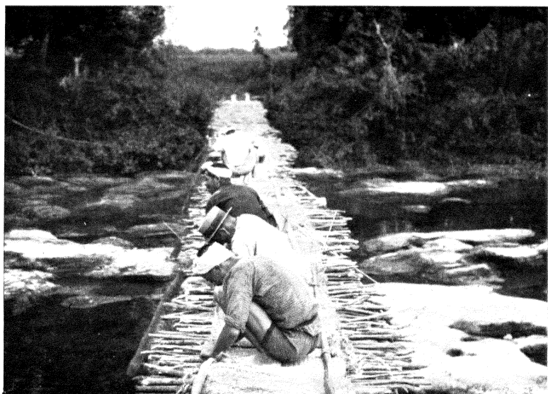
CIVIC CO-OPERATION IN BRIDGE BUILDING (IMAMURA BURAKU)
