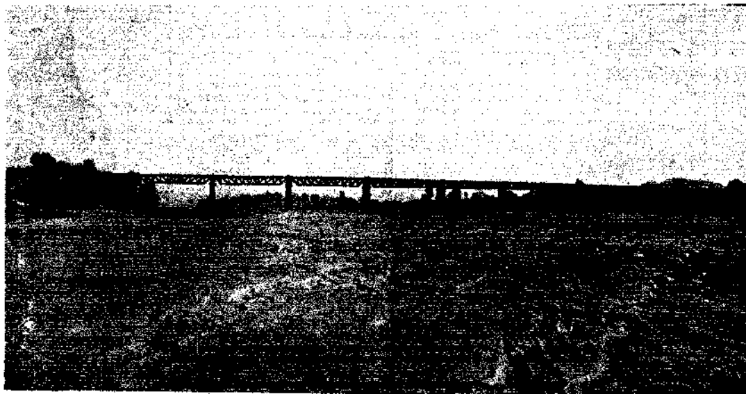
BRAHMINI BRIDGE I BETWEEN CHAKARDHARPORE AND JHARSUGUDA.
