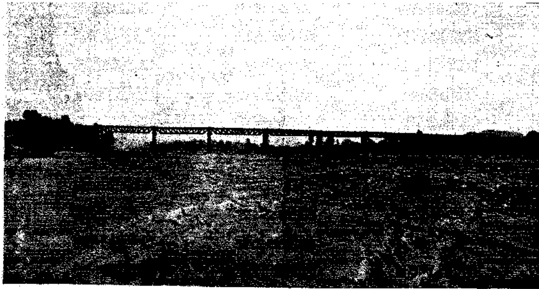
BRAHMINI BRIDGE: BETWEEN CHAKARDHARPORE AND JHARSUGUDA.
