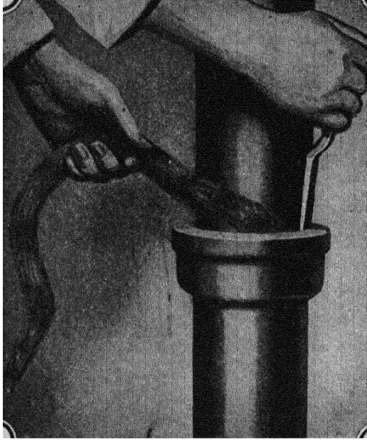
FIGURE 18-2.—Yarning the oakum in a joint.
