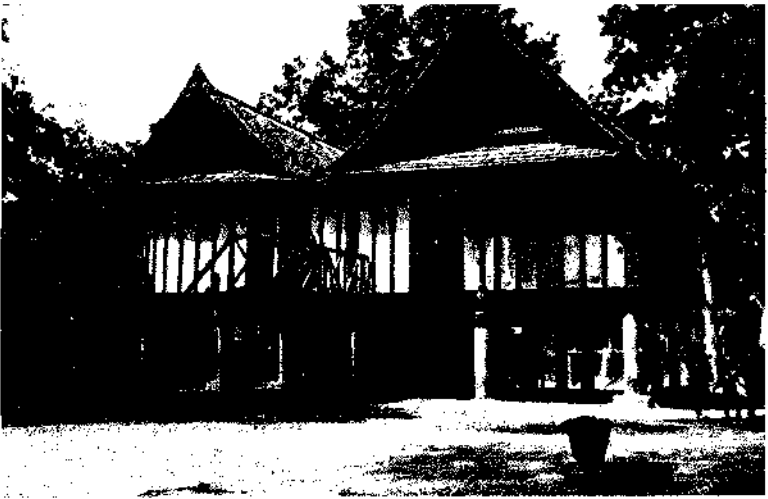
Teak bungalows built seven feet off the ground to withstand floods.
