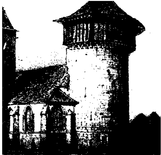
FORTIFIED CHURCH IN BURGUNDY XVTH CENTURY
